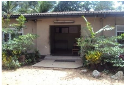
Figure 9: Selected brick work building
