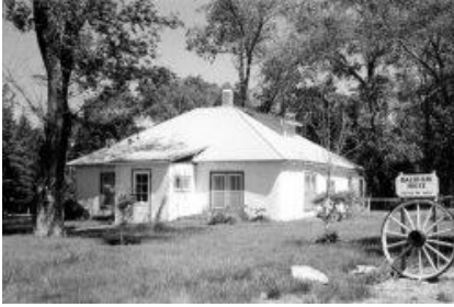
Figure2: Hay-bale house built in Nebraska in 1925 [11]
