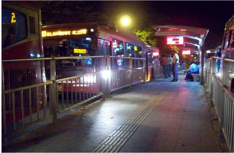
Fig. NO. 8: Accessibility to BRT on Surface Street in Delhi
