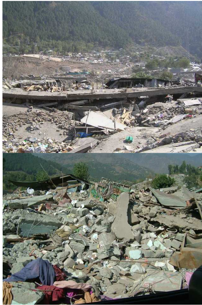
Figure 2: Major destruction due earthquake at Balakot City
