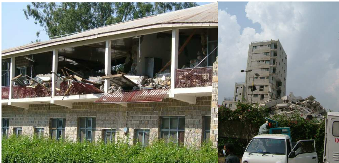
Figure 3: Destruction due earthquake at Islamabad and Abbottabad
